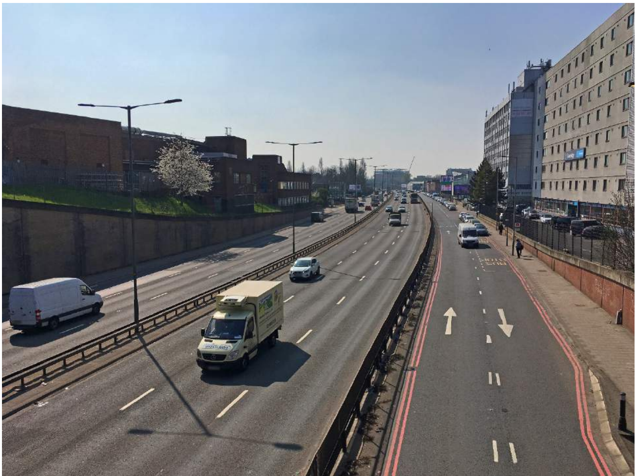
Figure 14. A stretch of pavement (looking north east), less than 100 yards in length, adjacent to the A406 between Priory Gardens and the bridge carrying the Uxbridge branch of the Piccadilly line (top); more than half a mile of minor road adjacent to the A406 (looking south west) – confusingly called the 'North Circular Road' – stretching from the bridge to the North Circular Aquaduct (bottom).
