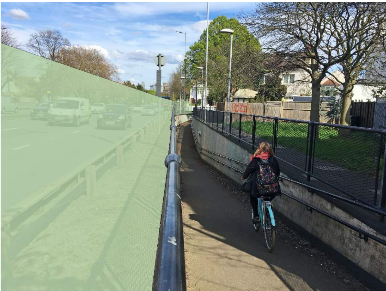
Figure 28. Looking north east along access to underpass to the south of Great West Road, close to the junction with Netheravon Road South, pictured as it is at present (top) and with proposed GI4RAQ (bottom); the latter is only illustrative, and TfL's arboriculture team should be consulted on all planting.
