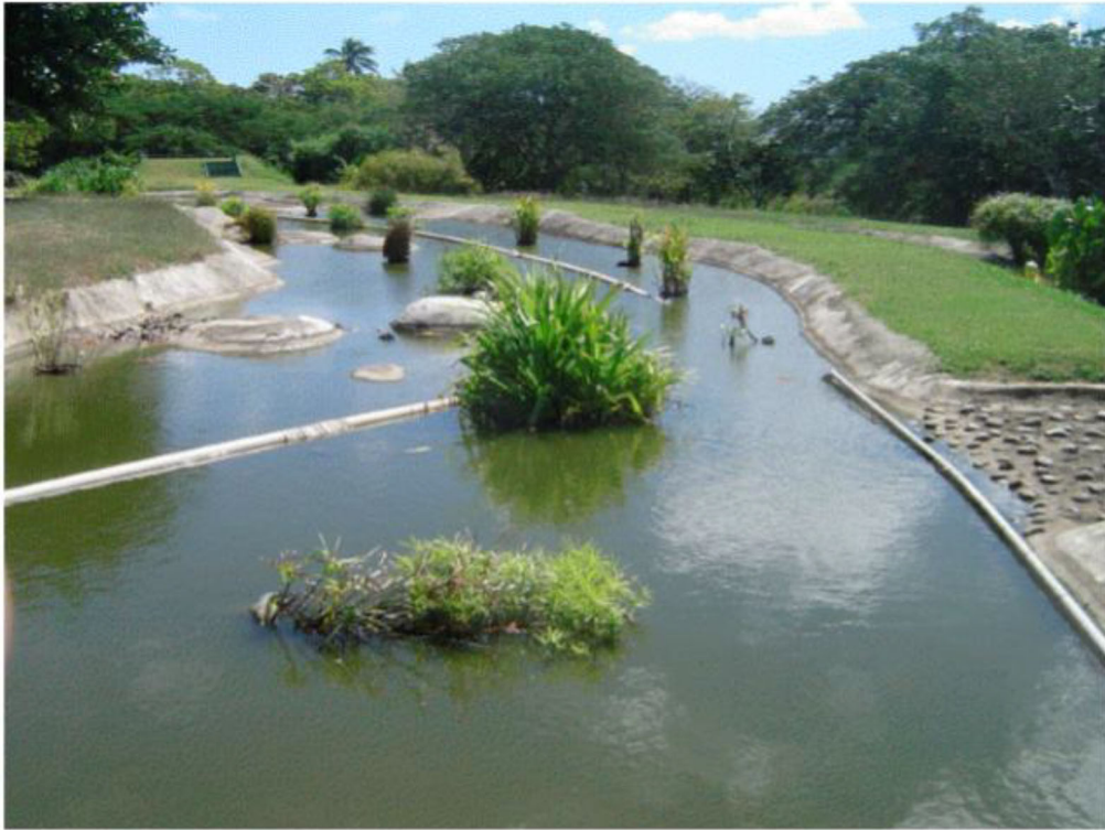
Figure 3. One of a series of three surface-flow constructed wetlands set up in Tangage village, on the Coral Coast of Fiji to receive treated wastewaters recirculated from the adjacent irrigation water storage pond (Photo: Chris Tanner).
