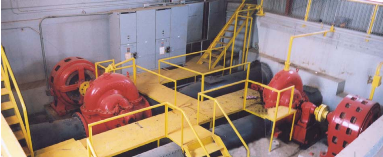
EXHIBIT C2. Two 45-cfs Pumps with Motors, Brownsville Irrigation District Rio Grande diversion pumping station, 2003.
