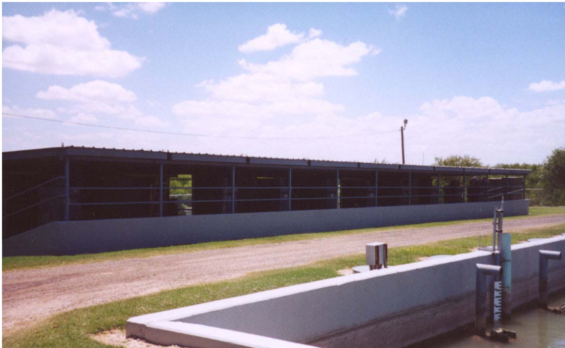
EXHIBIT C4. Back View of the HCID2 Pump House, 2003 (Stubbs).
