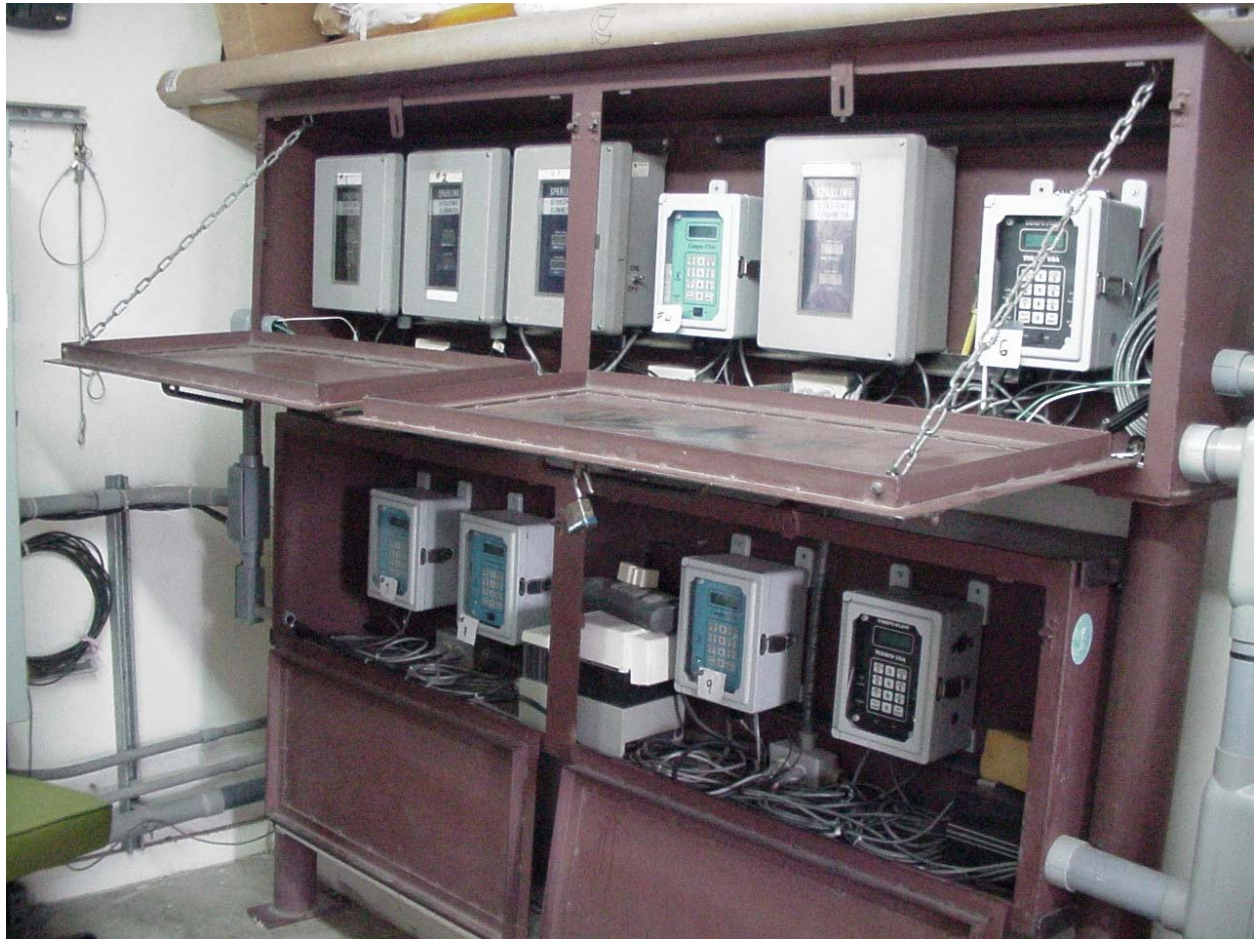
EXHIBIT C7. HCID2s Pump House Meter Recorders Used by the TCEQ Watermaster, 2004 (Hinojosa).
