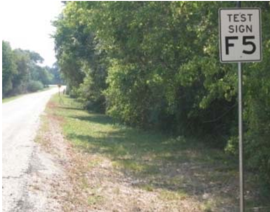
Figure 20. Example of Test Sign on Silver Hill Road
