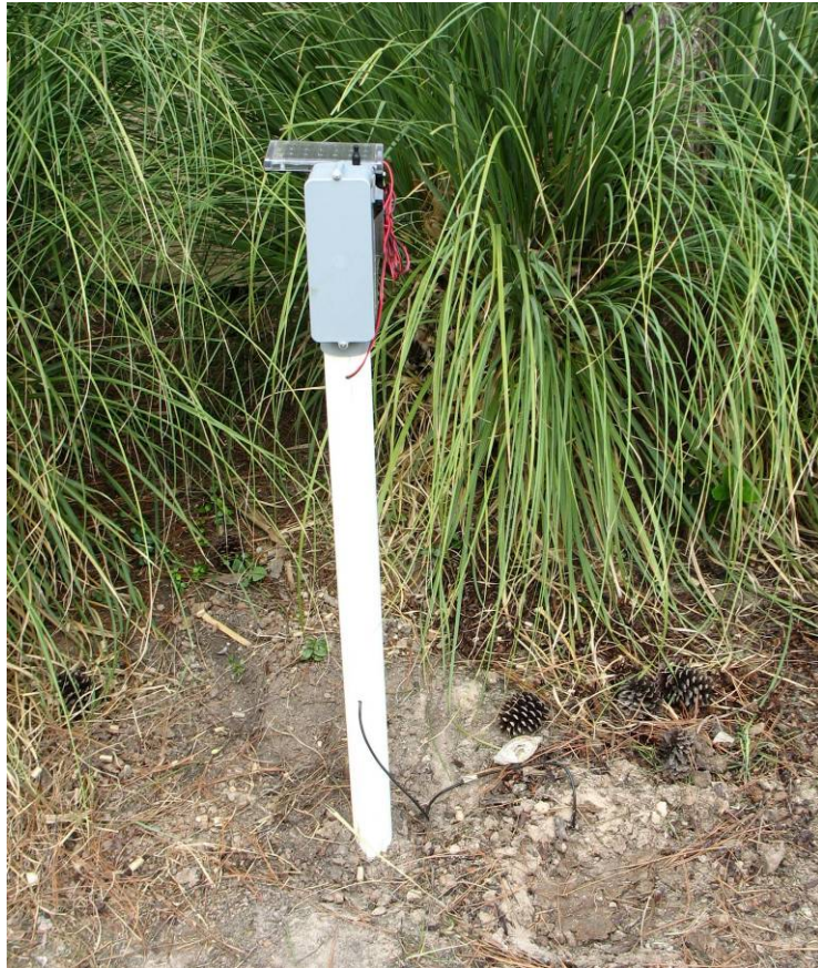
Figure 20. Trial 2 field installation of sensor node.
