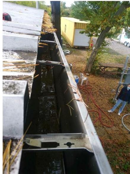
Figure 23. Canopy Roof Conditions. The figure on the right shows the gutter guard removed on a section for the photo, to see the pine needles that passed through.
