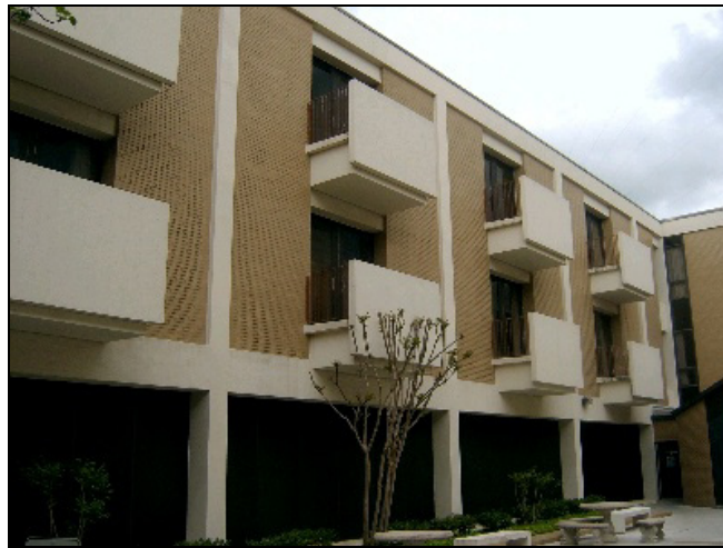
Figure 49-Exterior view of St. Joseph Regional Health Center.
