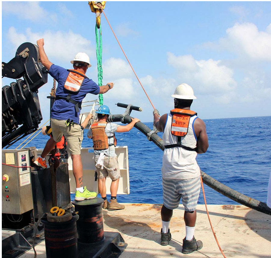
Figure 9. NTAS-19 EM chain deployment. The crane lifts the EM chain over the port rail with the buoy still in place on the deck.
