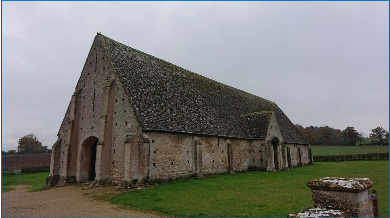
Figure 2 This impressive barn at Great Coxwell built c. 1230 features a typical layout for medieval barns seen across Britain. Two porches sit centrally opposite one another, with the east porch (visible, right) slightly higher on the incline than the west porch (not visible). The gable end entrance (visible, left) was added later to accommodate larger carts and machinery. Plenty of putlog holes can be seen along the length of the barn and at the gable ends. Photo: author.
