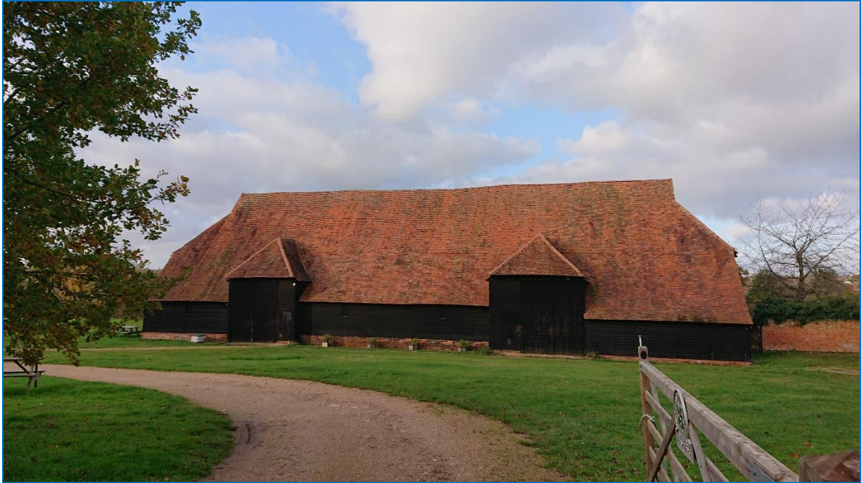
Figure 10 The Grange Barn (built to store produce farmed from an outlying grange) at Coggeshall is located above and at the edge of the present-day village. It would have also stored tithes for Coggeshall Abbey. It was built c. 1240 to a high standard, with both its size and position intended as an expression of wealth, despite the abbey itself accumulating significant debt. Photo: author.
