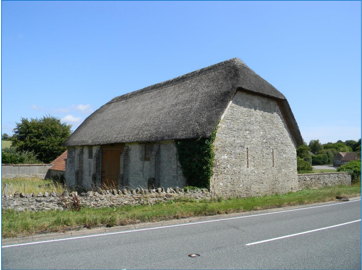
Figure 1 The 'Tithe Barn' at Whitcombe, Dorset dates from the 18th century by which time the farm was no longer owned by the Church. Though tithe payments were made to private landowners, particularly following the Dissolution of the Monasteries in the 16th century, there is little evidence to suggest that this barn ever stored tithes. Despite this, the barn is frequently referred to as 'The Tithe Barn.'
