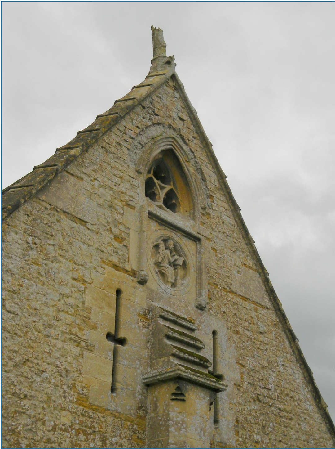
Figure 4 Much adorns both the interior and exterior of the Abbey Barn at Glastonbury built c. 1340. This barn stored produce farmed directly from the Abbey itself and so is not thought to be a tithe barn. The opening at the roof's apex is possibly an 'Owl Hole' though no proof for this as its intended purpose can be found. Photo: author.
