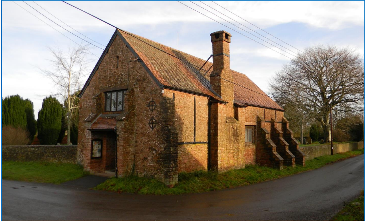
Figure 11 The 14 th century tithe barn at Fitzhead is still owned by the Diocese of Bath & Wells but is now used as a village community venue. The addition of a chimney and absence of some buttresses and cart entrances show that it has been some time since it was used regularly for agricultural storage. Photo: author.
