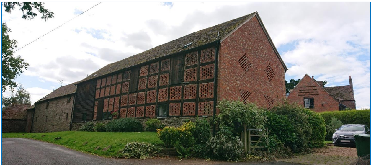
Figure 12 Tithe House at Stanton Long in Shropshire dates from around the 17 th century and features brick and weatherboarding rather than stone. It is now a private dwelling. Photo: author.
