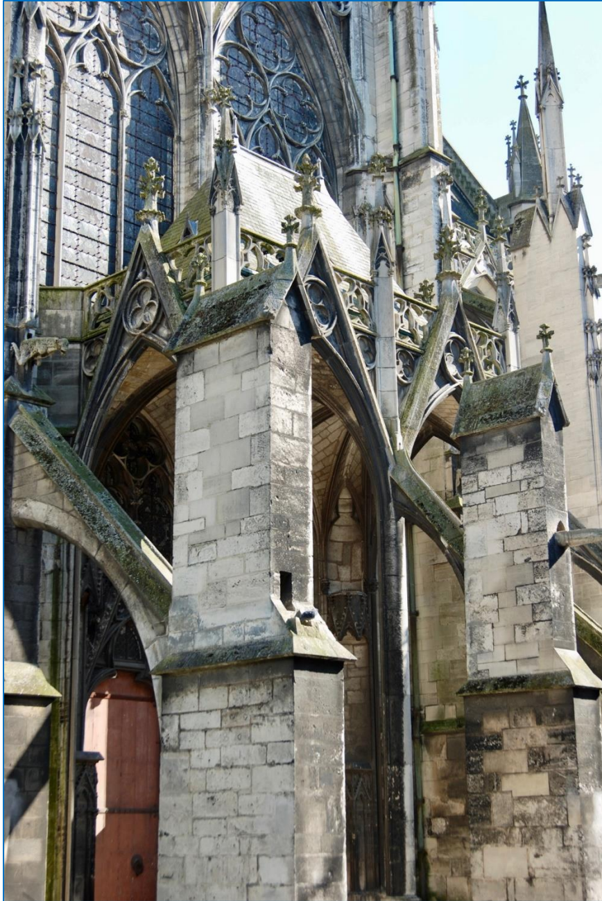
Figure 1 Troyes, Saint-Urbain, view of porch buttresses and flyers. Photo: author.
