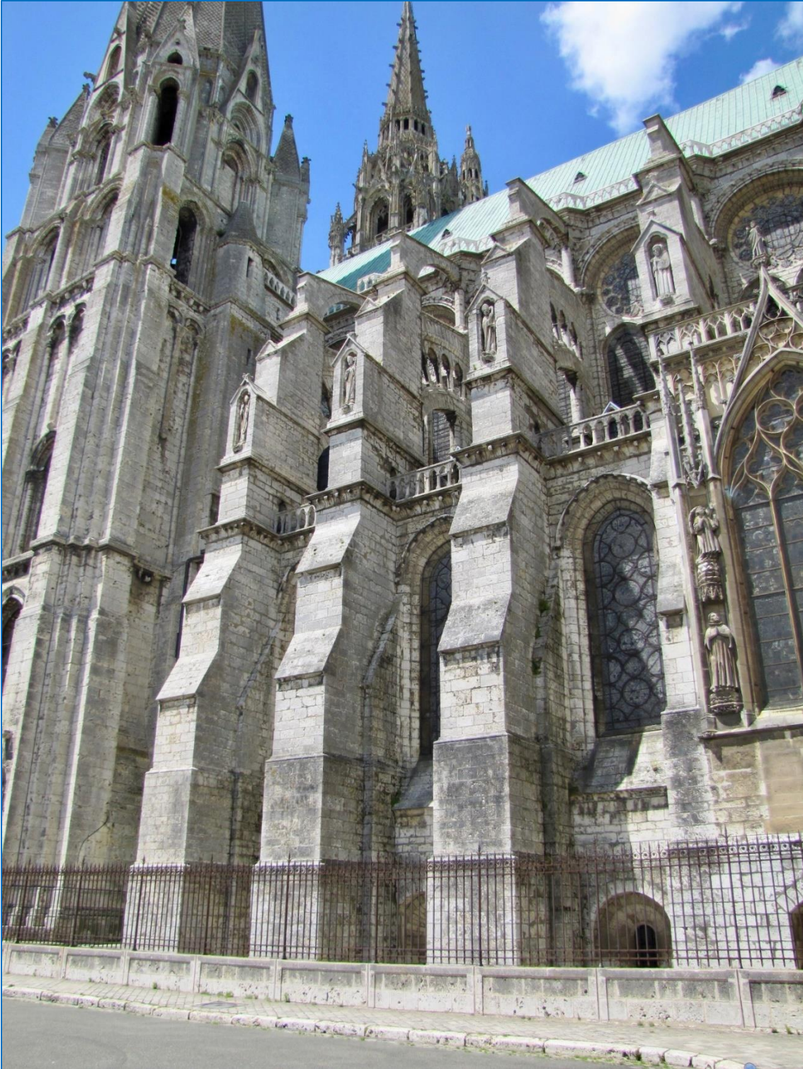
Figure 2 Chartres Cathedral, south nave elevation with buttress interstices. Photo: author.
