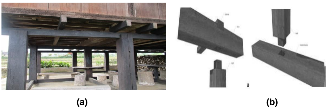
Figure 7. (a) The Joint Pole of Baghi/Besemah Traditional House and (b) Sako Pedestal on Foundation and Floor (Nasution and Prasetyo, 2016).
