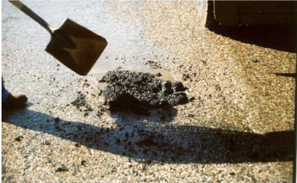
Figure 1.2. The throw-and-roll procedure – material placement (Source: [5])
