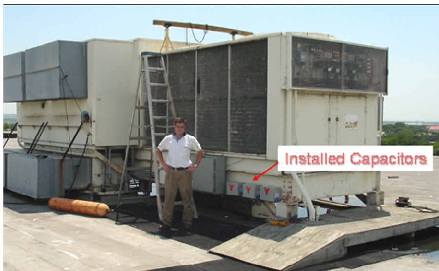
Fig. 25. Installed capacitors
