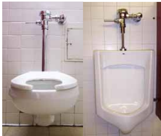
Figure 2. Manual low-consumption water closet and urinal (Hwang, 2003)
