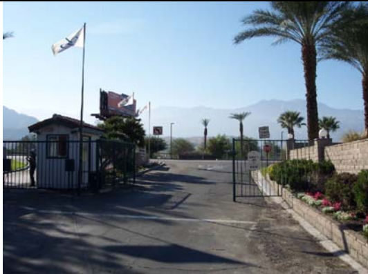
Figure 2.10: Gate and Guard House
