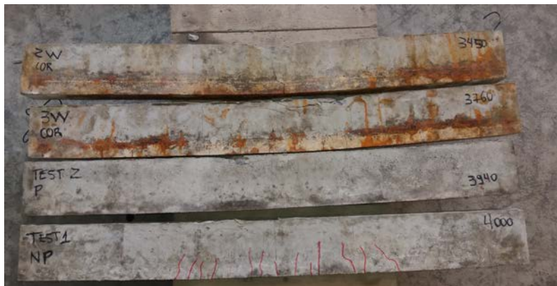
Figure 12 - Crack mapping of the CO and RE beams
