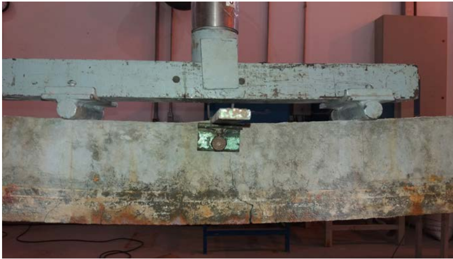
Figure 7 - Main crack in the pure flexural zone of beam CO 14%
