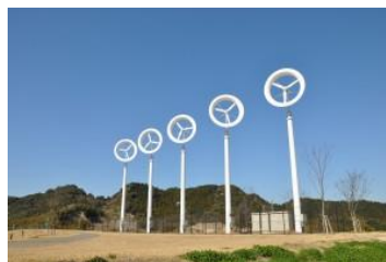
Fig. 1-5 Wind farm of wind turbines with a brimmed diffuser at Kyushu University [11].
