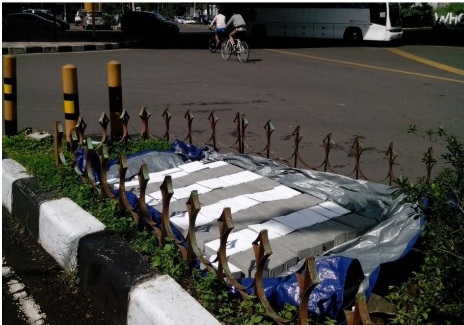
Figure 2 Placement of paving blocks coated with \text{TiO}_2 on Juanda Street in Bandung City. (Source: research documentation)
