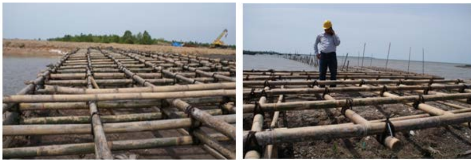
Figure 5 Gridded Matress Bamboo for Soft Soil Reinforcement.
