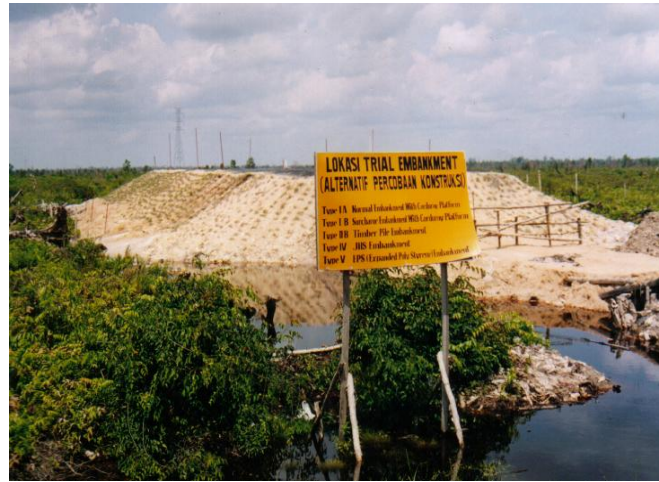
Figure 9 Trial Embankment Construction [1].
