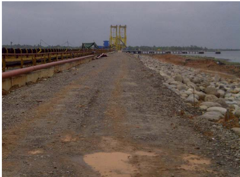
Figure 7 Causeway embankment after construction in Pangkalan Susu.
