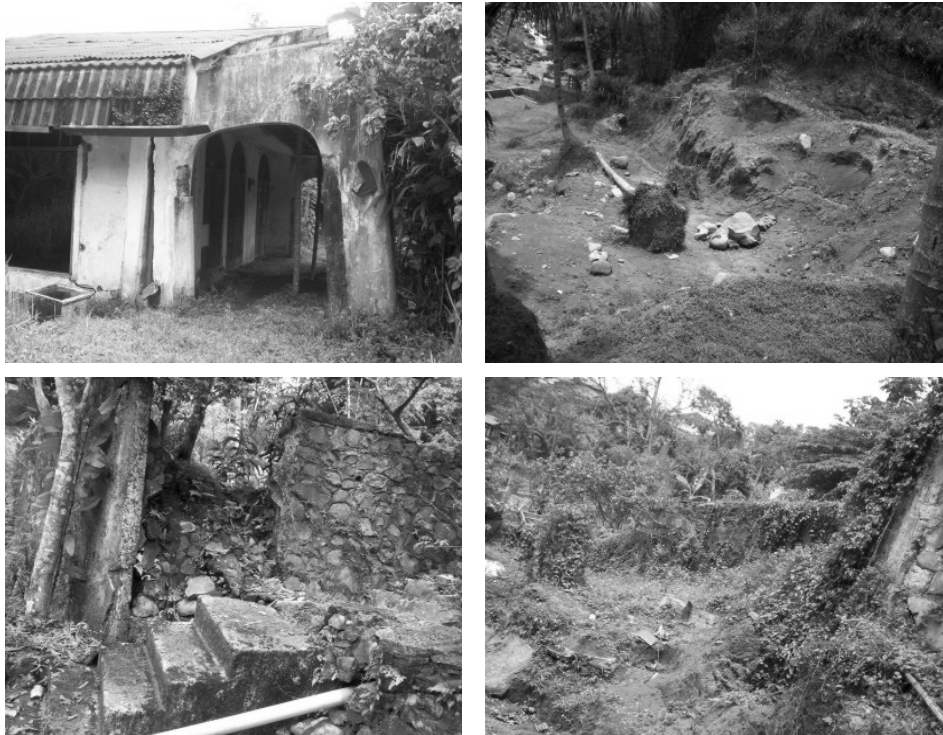
Figure 2 Example of landslide impacts in Megamendung.
