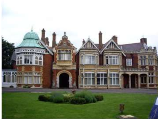
(a) Main building
