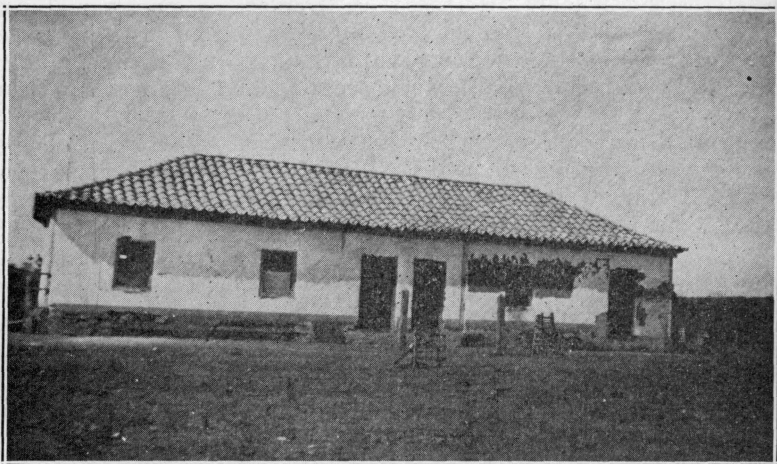
Figure 25. Tenant House in Interior of Central Brazil. Brick with Tile Roof. (Photo, courtesy Professor T. R. Day, 1922.)
