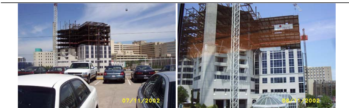
Figure 3.14: East Link Tower, Children's Expansion Project
