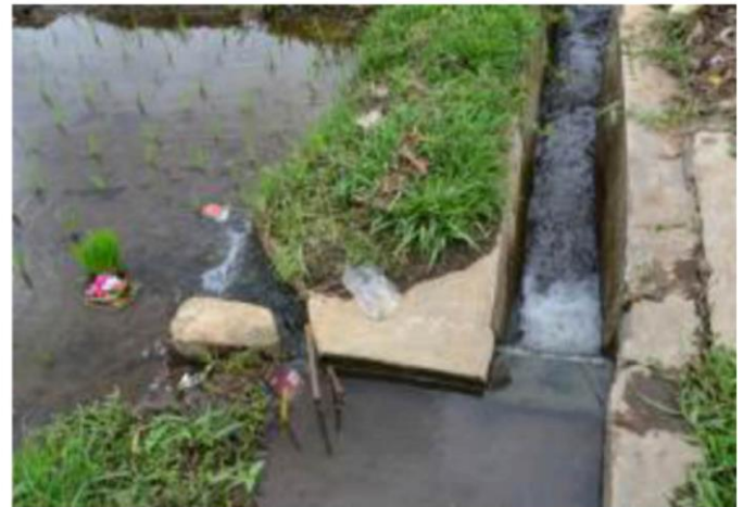
Figure 1 Typical water distribution unit ( tektek or kecoran ) in water flow on a continuous basis
