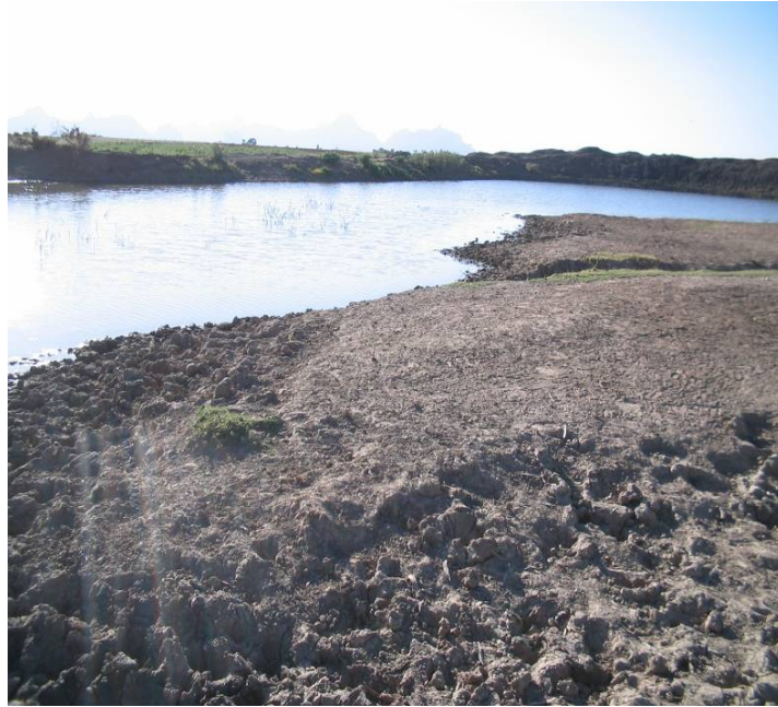
Figure 4.1. Percolation ponds constructed in the watershed.
