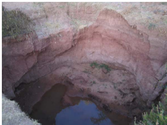
Figure 4.3. Sliding of the walls in hand dug wells in the watershed.
