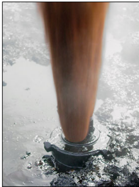
Fig. 5.1 –South Rumalia Well RU-67 flows vertically after production head removal, pre-sting and kill operation. 11
