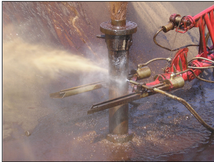
Fig. 5.2 – Hydra-Jet cutter cutting below wellhead with gelled sand/water slurry. 44
