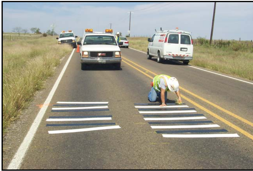
Figure 6. Installation of Rumble Strips
