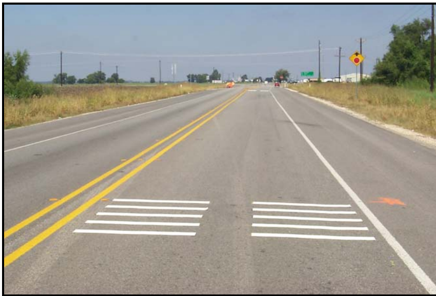
Figure 7. Upstream View of Installed Rumble Strips
