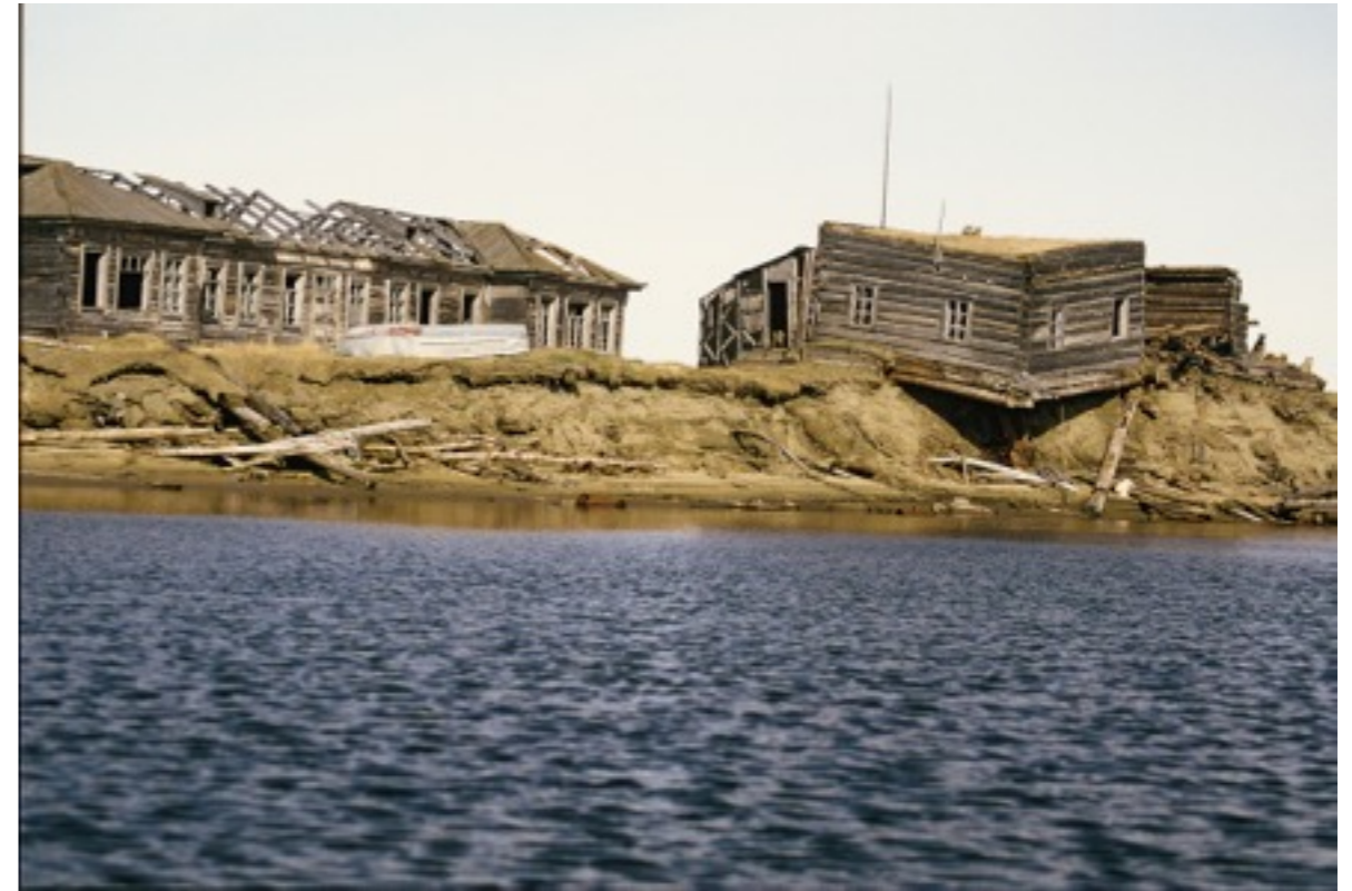
This picture is taken in Siberia of a former Stalin camp. The remnants are collapsing due to permafrost thaw.
