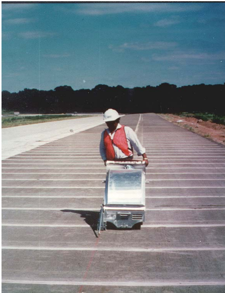
Figure 2-1 Timing of sawing contraction joint is critical.
