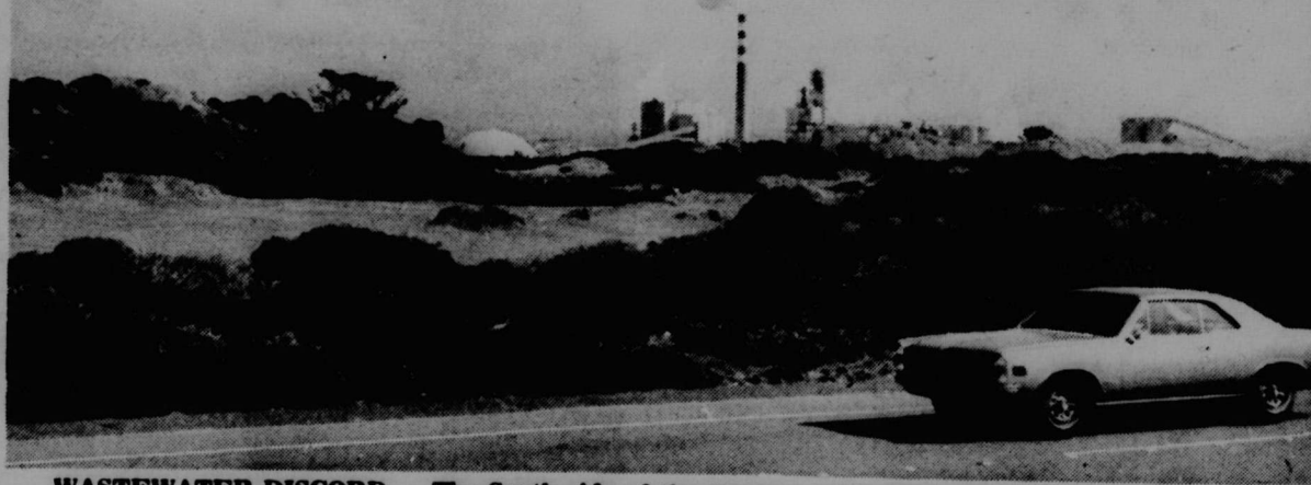
WASTEWATER DISCORD — The South side of the Samoa peninsula is the proposed site for the Humboldt County marsh reclamation sewer project.
