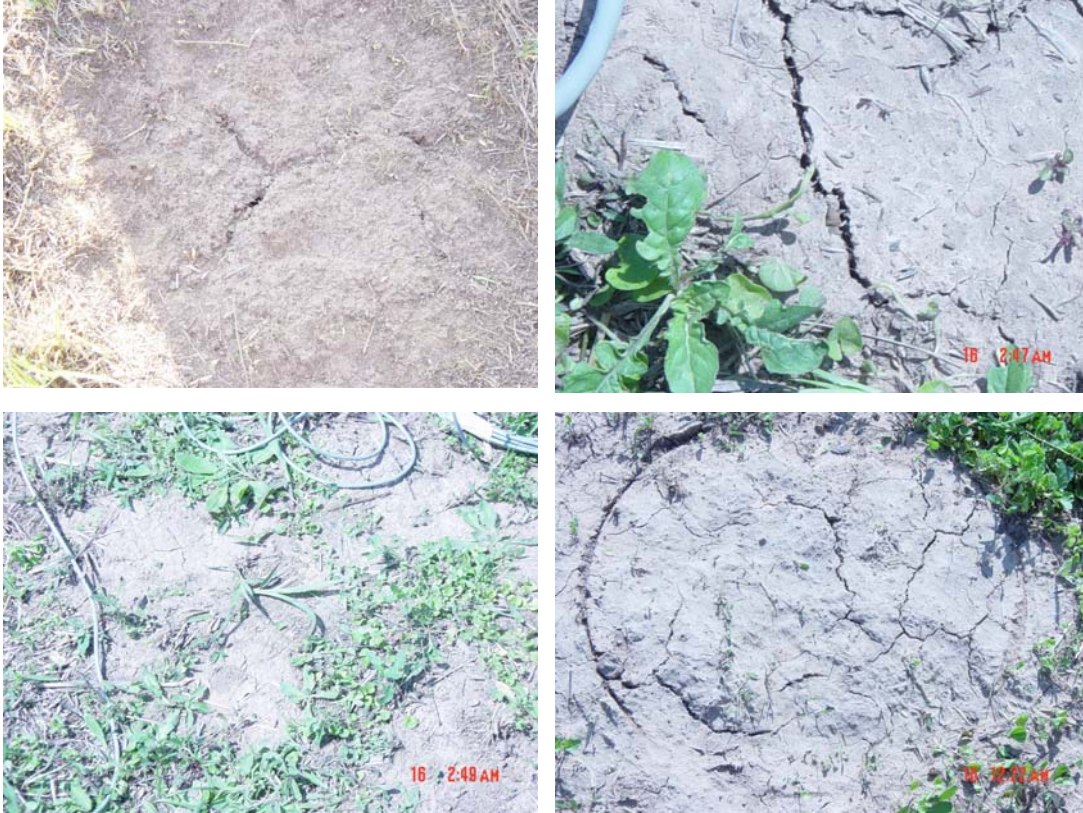
Fig. III-2. Vegetation and surface cracks in soil within the experimental plot.
