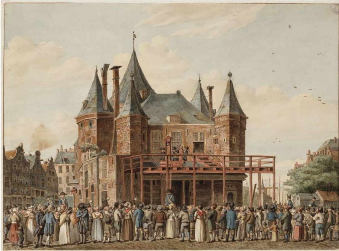
fig.14: Gerrit Lamberts (1812) Guillotine poor de Waag
