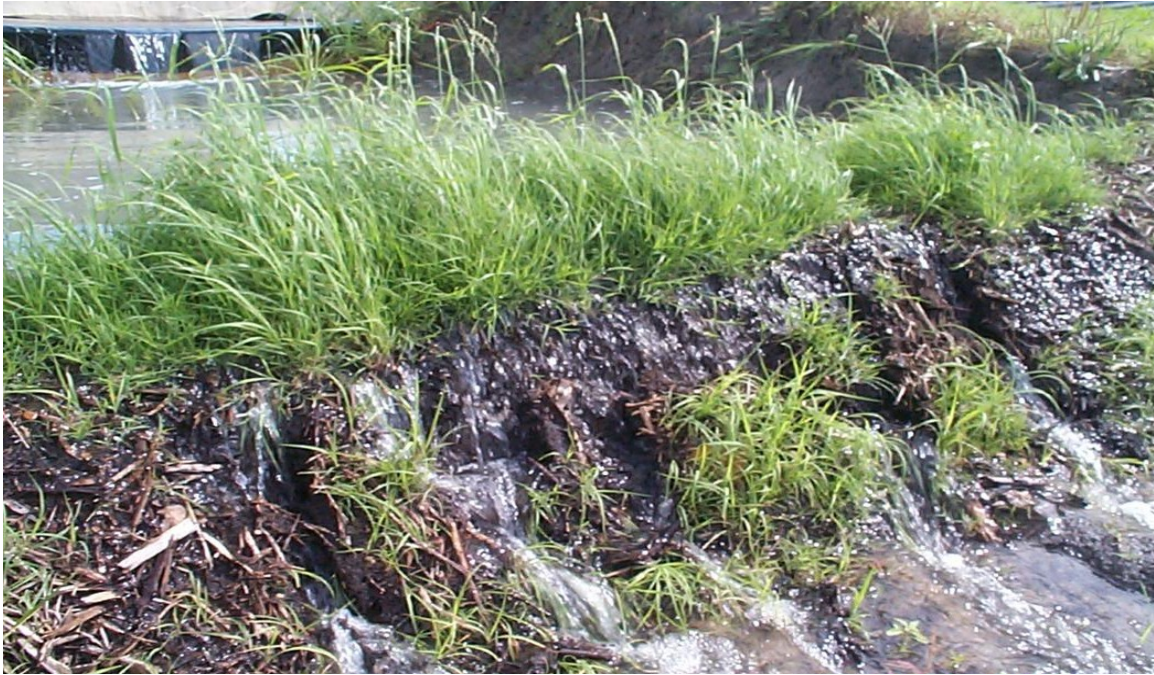
Figure 5.40 Dairy manure compost berm showing minor damages to the leading face.
