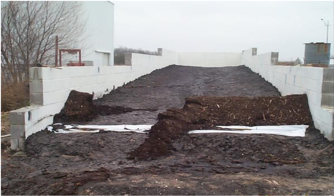
Figure 5.1 Failure of the berm on clay soil due to displacement.
