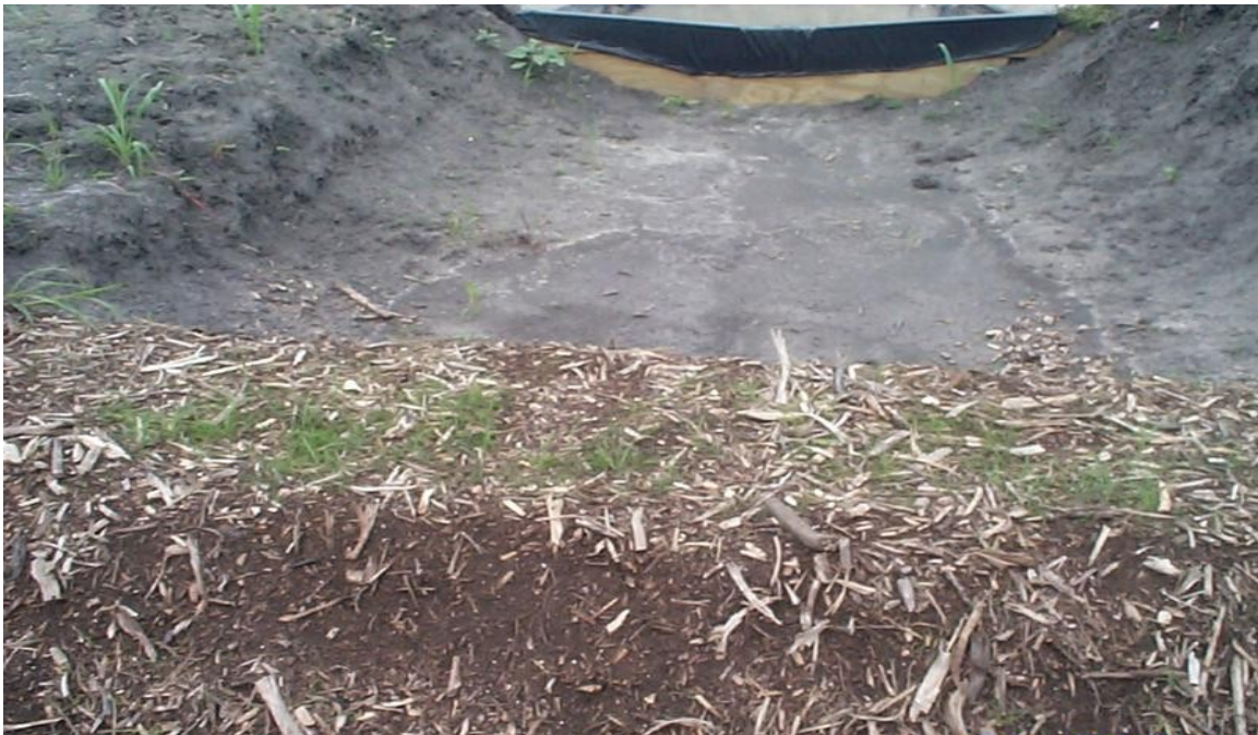
Figure 5.36 Composted bio-solids berm before starting the structural testing.
