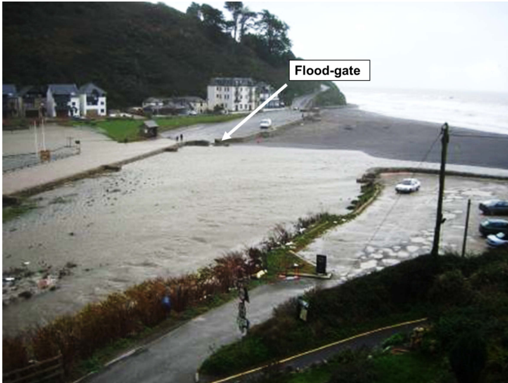
Figure 2.5: Seaton beach, Cornwall, 2006, the flood gate remains open during the flooding event (@NFDC)
