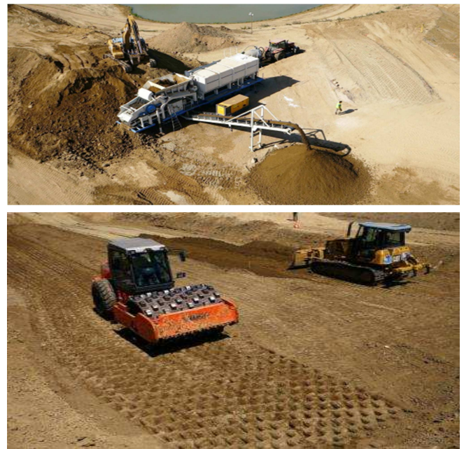
Figure 4. Experimental dike after completion of the construction steps.
