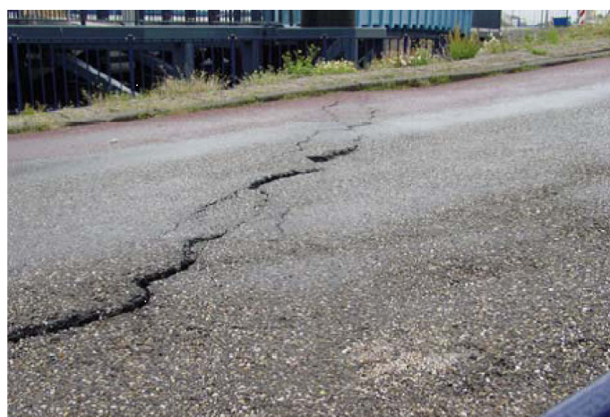
Figure 1. Damage induced by a propeller jet at a quay wall.
