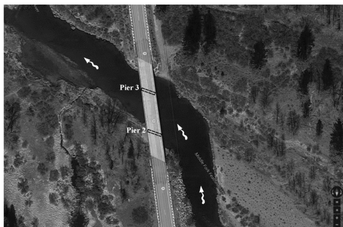
Figure 1 Bridge Site on State Route 89 over the Middle Fork Feather River CA, USA (Source Google Maps 2016).
