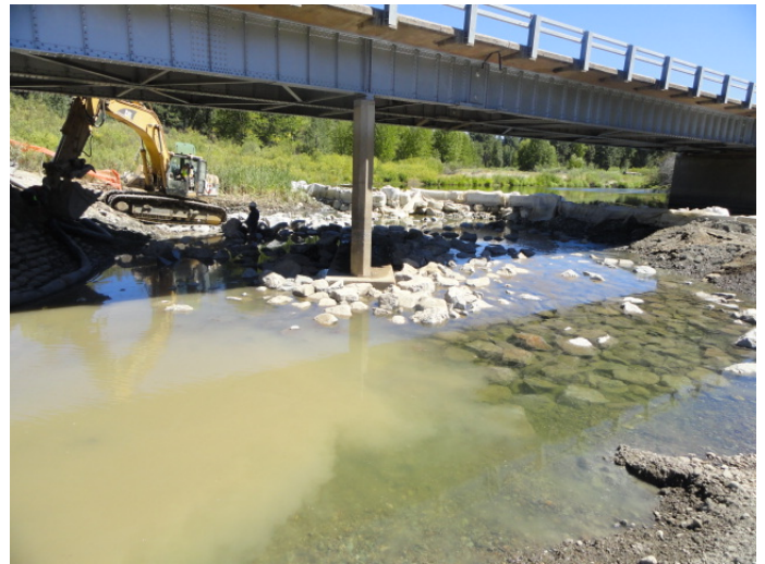
Figure 2 Riprap installation around Bridge Pier 3 at the Middle Fork Feather River
