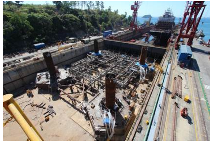
Figure 2. Truss-linked pad footing foundation system under construction
