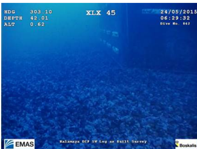
Figure 12. Pad footing placed upon seabed preparation
