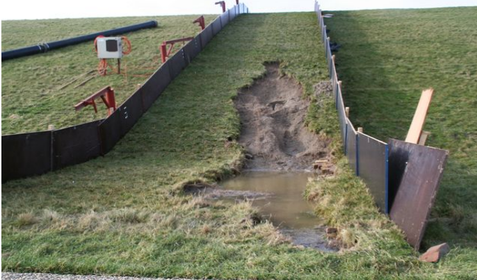
Figure 3.5 Geometrical transition (at toe of dike)
