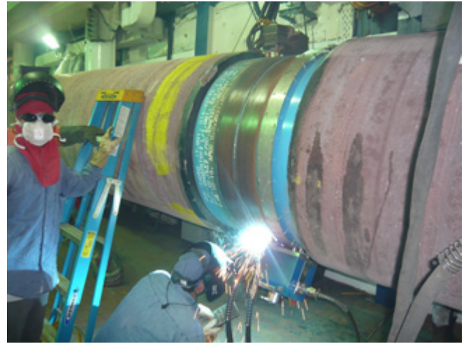
Figure 4 Example of Offshore Pipeline Welding (Lincoln Electric, 2015)
