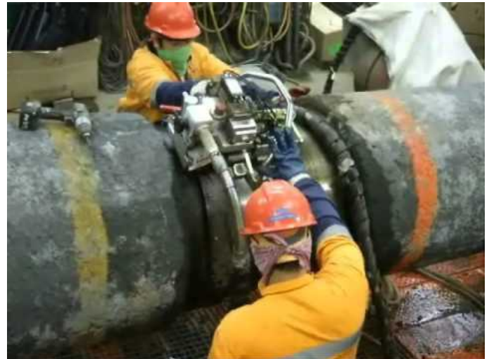
Figure 5 Example of Offshore Pipeline NDT (Rörvik, 2011)
