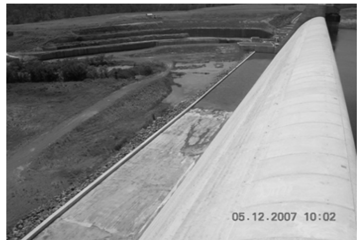
Figure 1. View of primary spillway of Paradise Dam
