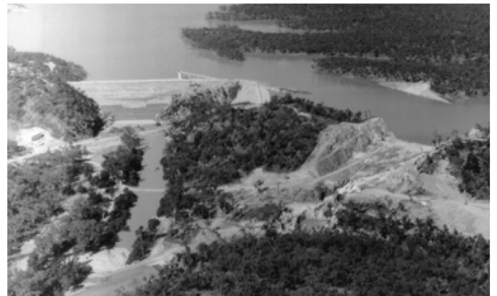
Figure 7. Aerial view of Boondooma Dam (left) and of unlined discharge chute (right)
