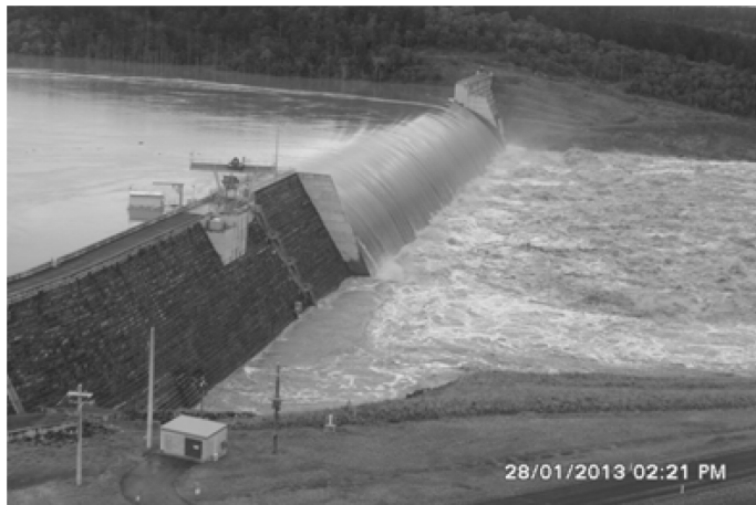
Figure 3. 2013 flood at Paradise Dam primary spillway
