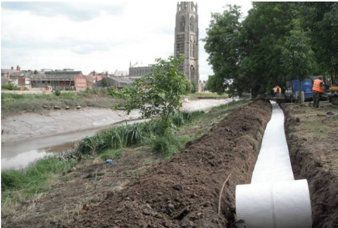
Figure 2: Installation of GeoDetect fibre optic cable in geotextile mat
