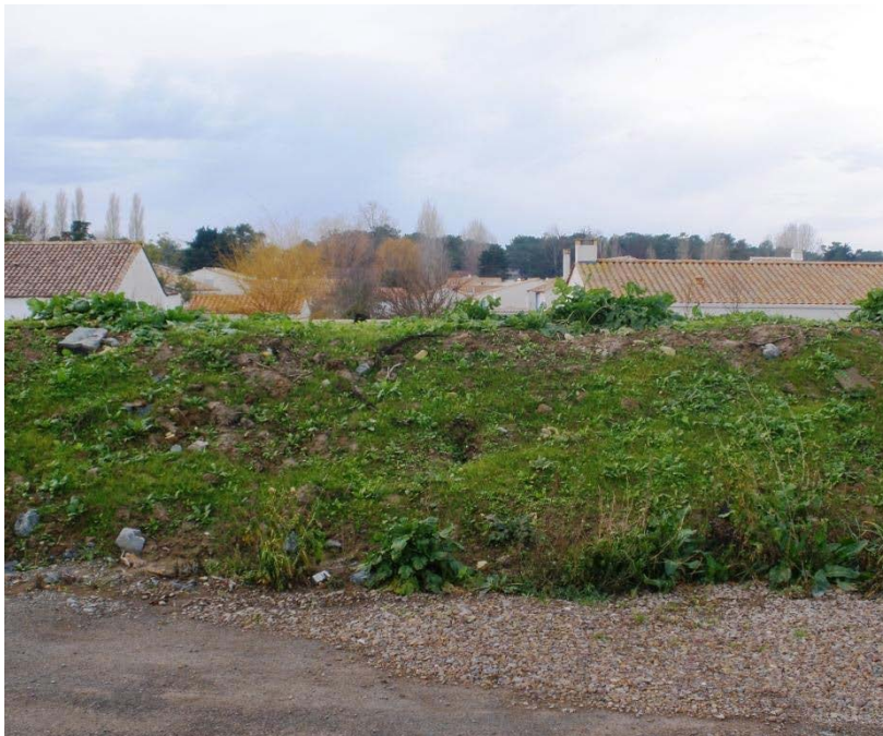
Figure 7: Single storey houses located behind coastal flood defences in La Faute-sur-Mer
