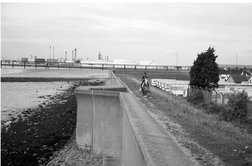
Figure 10: Improved flood defences built to protect Canvey Island following the 1953 flood
