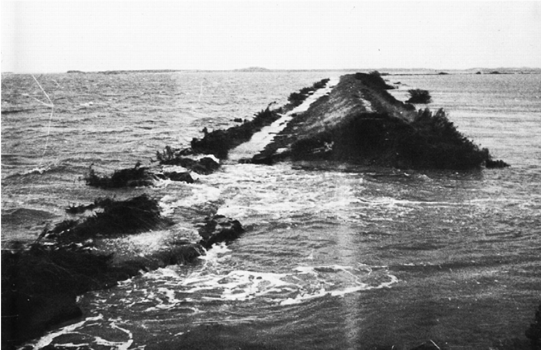
Figure 2: Typical breach in the flood defences during the 1953 floods
