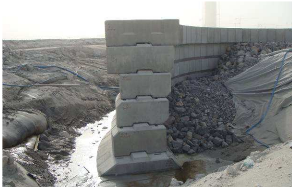
Blockwork wall (Halcrow)
