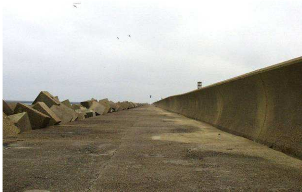
Crown wall on rubble mound breakwater (CETMEF)
