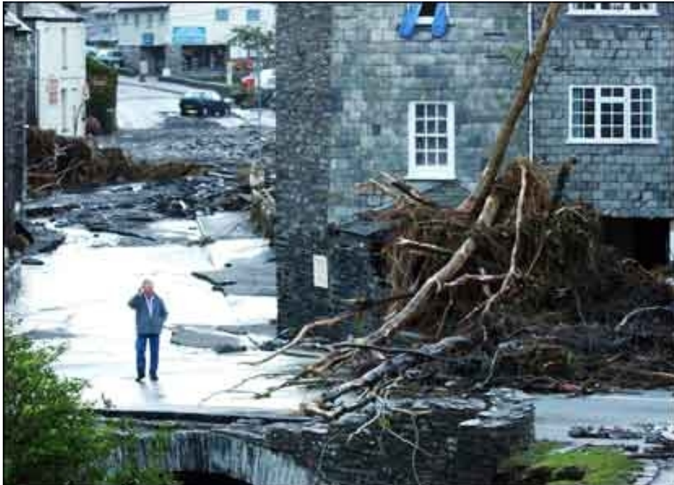
Plate 6.4 Photograph showing debris against the upstream parapet of the B3263 Road Bridge. Source: BBC
