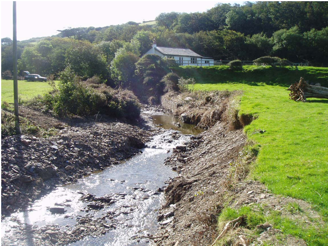
Plate 6.5 Conditions 500 metres upstream of bridge 1
