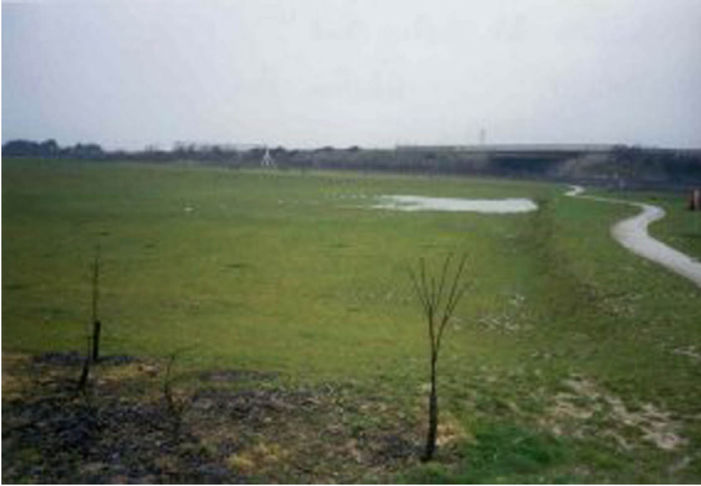
Figure 7 Brookfields Park detention pond
