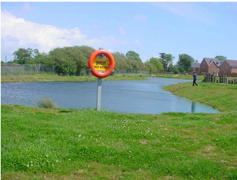
Figure 6 Brookfields Park retention pond
