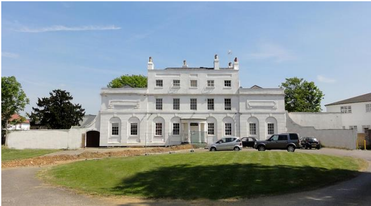
FIGURE A-6: WORTON HALL, ISLEWORTH, WEST LONDON STILL OWNED WITHIN THE CERF FAMILY WAS A 40 ROOM MANSION ORIGINALLY BUILT IN 1783 BY RICH MERCHANTS AND BECAME THE ISLEWORTH FILM STUDIO.
