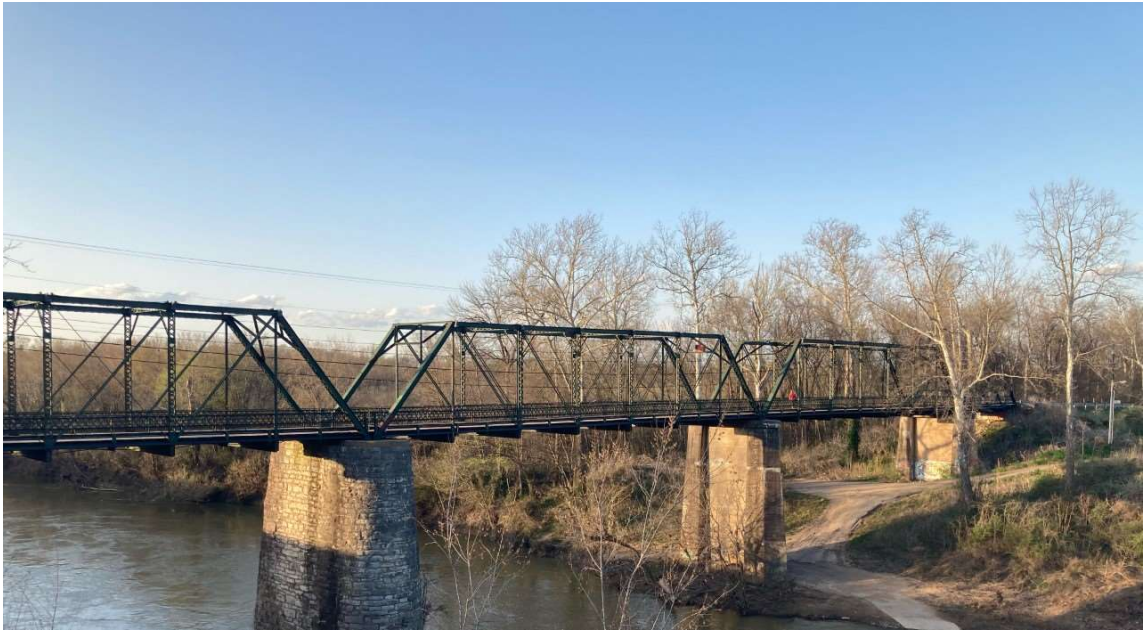
Figure A-1: Example of truss bridge
