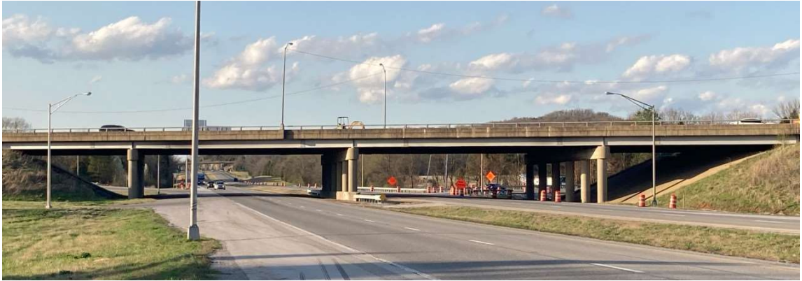
Figure A-3: Example of a beam bridge
