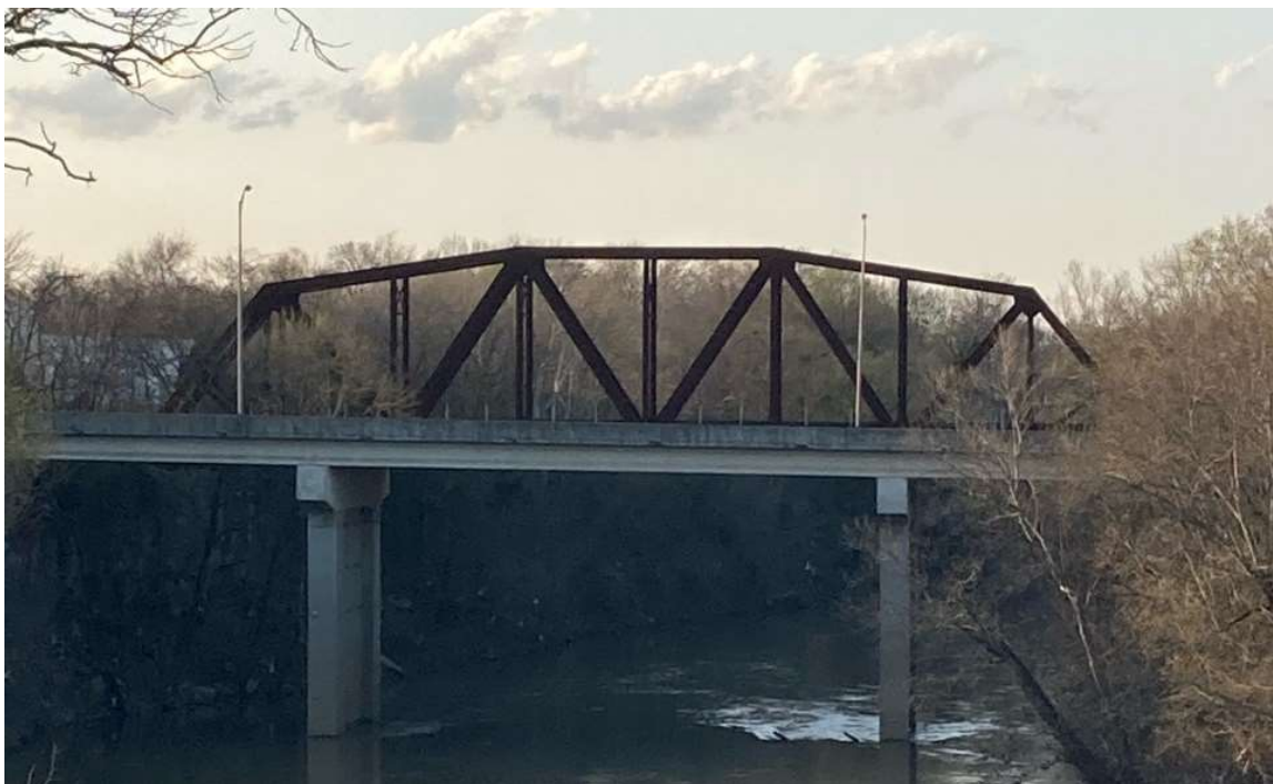
Figure A-2: Example of truss bridge
