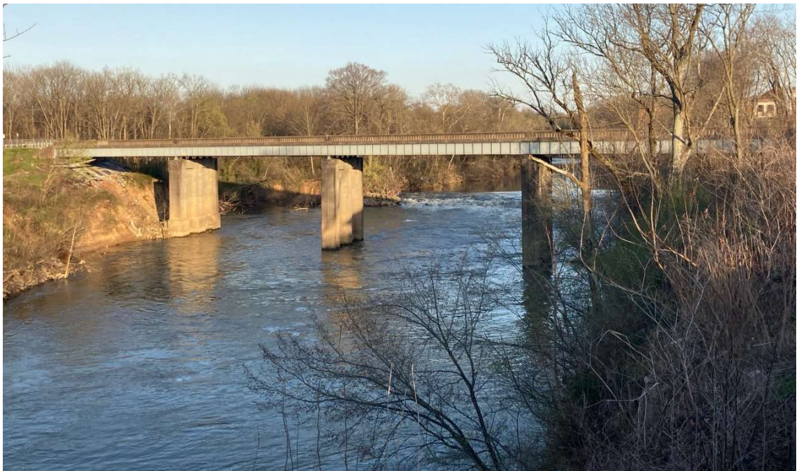
Figure A-4: Example of a beam bridge
