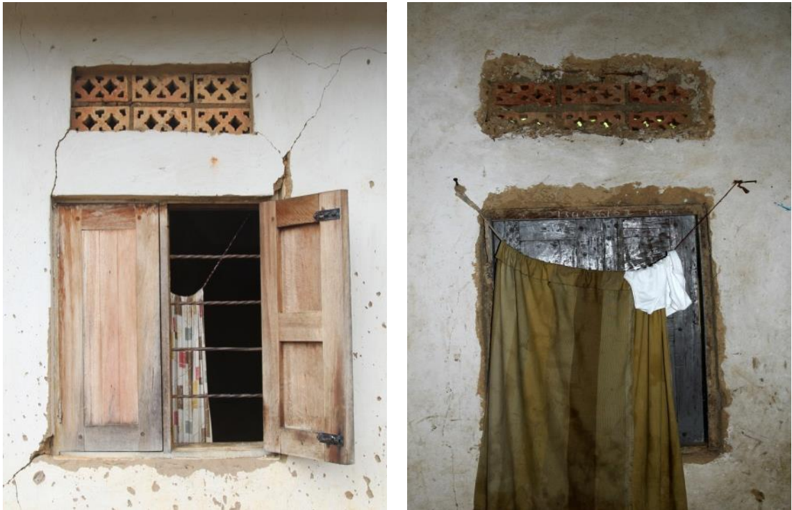
Figure 5.2. External (left) and internal (right) view of unscreened airbricks in Uganda
